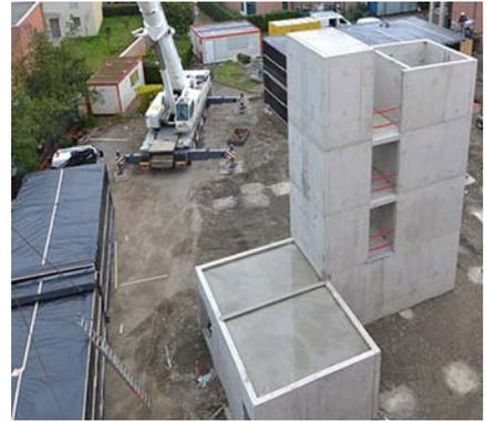
Construction process of the concrete cores. Stora Enso <https://n9.cl/z4k1e>
