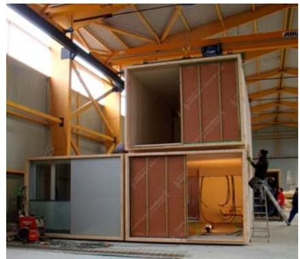
Workshop assembly of the prefabricated timber modules. Plataforma Arquitectura <https://n9.cl/56zq0>
