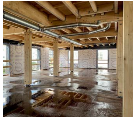
First floor structure phase. Timber posts and beams.
