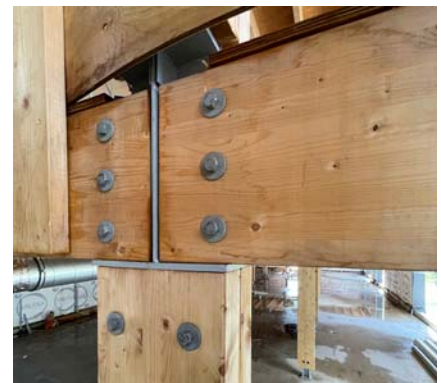
Post and beam joint.
