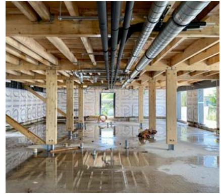
Basement floor construction process. Timber posts, beams and bracings.
