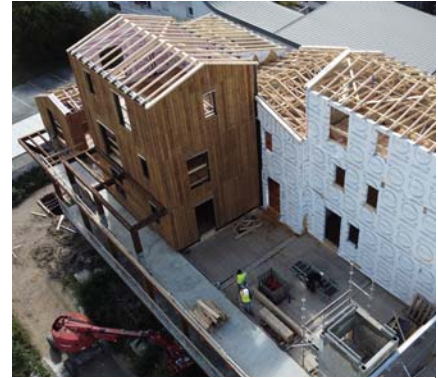
Construction process. Aerial view.
