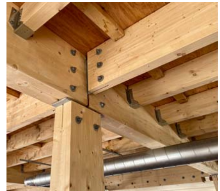
One-way slab with timber beams and joists.
