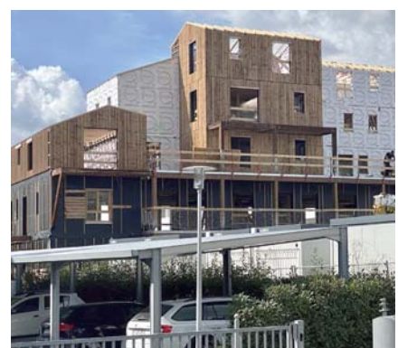
Main façade under construction.
