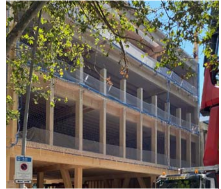
Construction process seen from the outside. Lacuna street.
