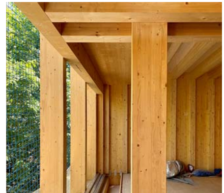
Joint of the GLT post with the CLT slab.
