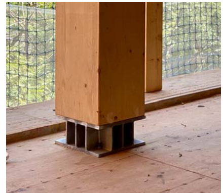
Joint of the GLT post with the CLT slab.
