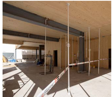
Steel posts and beams on the basement floor holding CLT panels.
