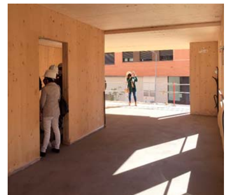
Construction process. CLT panels seen from a balcony. DiarideSabadell https://n9.cl/46tqo
