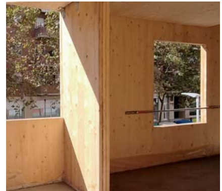
Construction process. CLT panels seen from a balcony. DiarideSabadell https://n9.cl/46tqo
