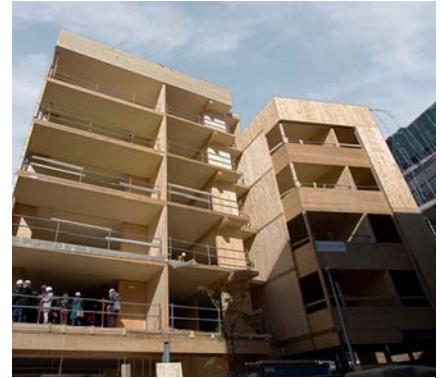
Construction process. Structural phase. DiarideSabadell https://n9.cl/46tqo
