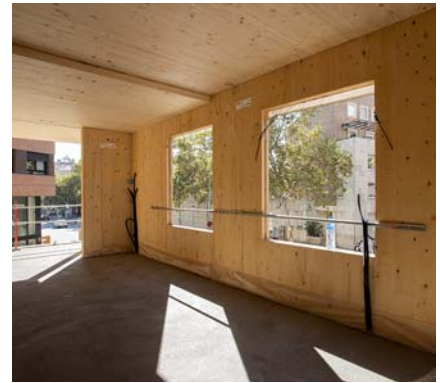
Construction process. CLT panels seen from de interior of a dwelling. DiarideSabadell https://n9.cl/46tqo
