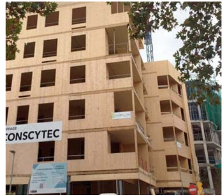
CLT panels on both Sabadell street and Barcelona road façades.
