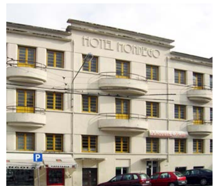
Construction process. Global Art Deco https://n9.cl/5192i
