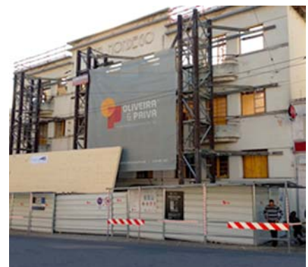
Exterior of the building.
