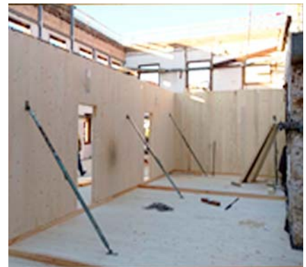
Construction process. Laying of CLT panels on interior walls.
