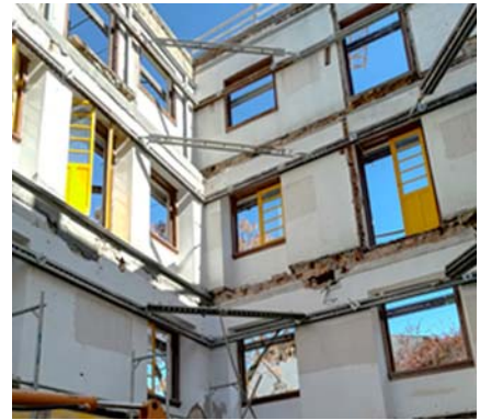
Art Deco façade after demolition process. TISEM https://n9.cl/d917x
