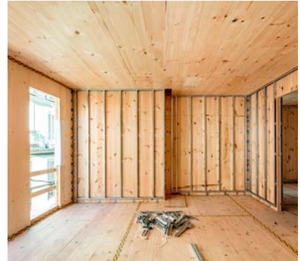
Construction process from the inside. Adrià Goula https://n9.cl/m2blt
