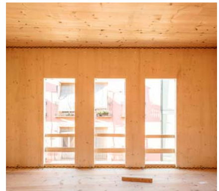
Building process. Exterior wall made of CLT. Adrià Goula https://n9.cl/m2blt
