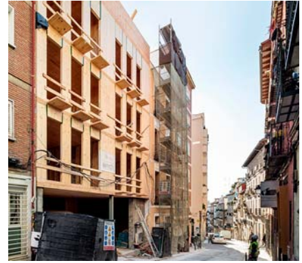
Buenavista Street during construction. Adria Goula https://n9.cl/m2blt
