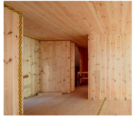
CLT panels used as walls and slabs. Adrià Goula https://n9.cl/m2blt
