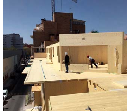
Construction process. Placement of CLT panels on the second floor.
