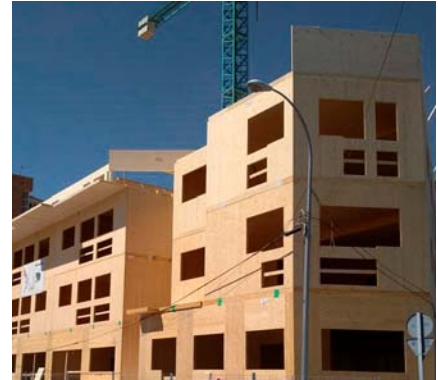
Construction process seen from the outside. Structure phase. Entrepatis https://n9.cl/vmzfc
