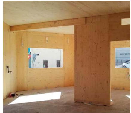
Construction process of the basement floor.
