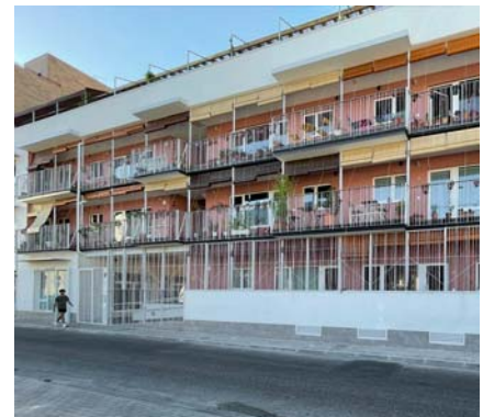
Main façade towards González Feito Street
