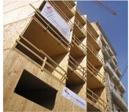
Construction process. CLT panels. Trass Arquitectura
