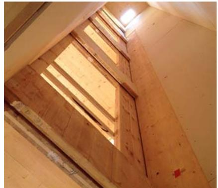
CLT core. Lift shaft. Trass Arquitectura
