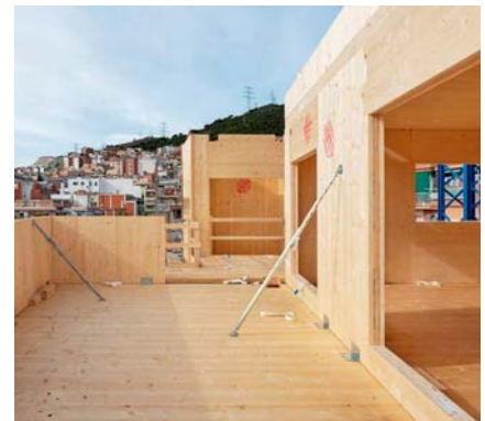
Terrace of the penthouses. CLT panel parapets, slabs and walls. CLT external walls and balcony overhangs
