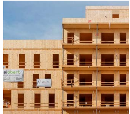
CLT external walls and balcony overhangs Guifré de Peray | Celobert cooperativa https://n9.cl/9ko3r
