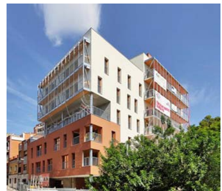
Port de la Selva and Pla del Cirerers street corner. Celobert cooperativa https://n9.cl/9ko3r
