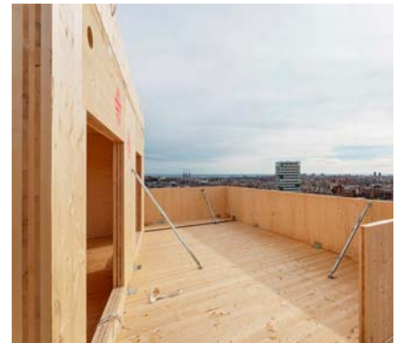
Terrace of the penthouses. CLT panel parapets, slabs and walls. CLT external walls and balcony overhangs
