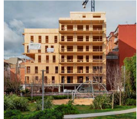
Construction process. Structure phase. Guifré de Peray | Celobert cooperativa https://n9.cl/9ko3r
