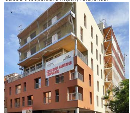
Pla del Cirerers street façade. Celobert cooperativa https://n9.cl/9ko3r
