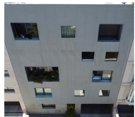
Aerial view of the entire façade.
