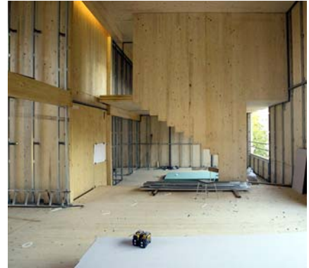
Construction process. 2nd floor apartment. Queima Films https://n9.cl/lgm3z
