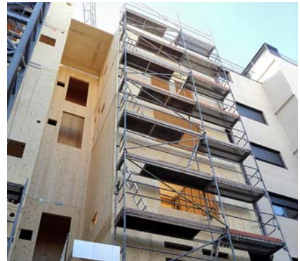
Back façade under construction. Madergia
