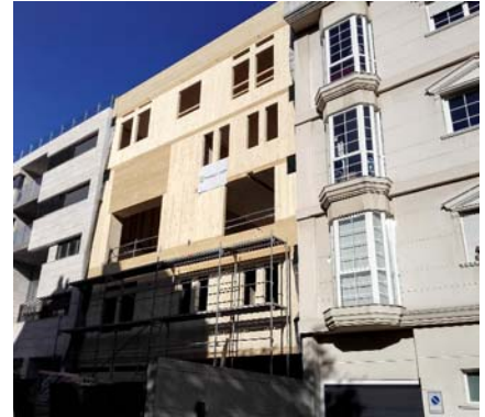
Main Façade under construction with CLT. Madergia
