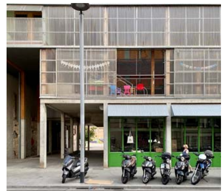
Ground floor and access to the building.
