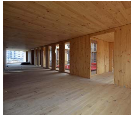
Construction process. CLT panels used in walls and floors. LACOL
