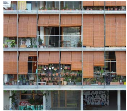
Detail of the back façade sunshades.
