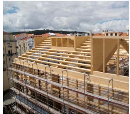
Construction process. Roof structure https://n9.cl/cv2z
