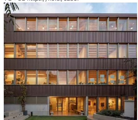
Inner courtyard FG + SG https://n9.cl/6256f
