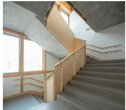
Concrete stairs core. FG + SG https://n9.cl/6256f
