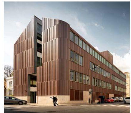
Northeast corner of the building FG + SG https://n9.cl/6256f
