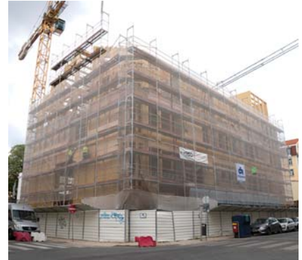
Construction process. Structure phase. https://n9.cl/cv2z
