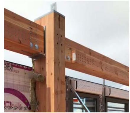
Detail image of the joint between timber posts and beams. Eiffage
