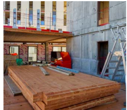
CLT floor panels stacked next to the reinforced concrete core. Eiffage
