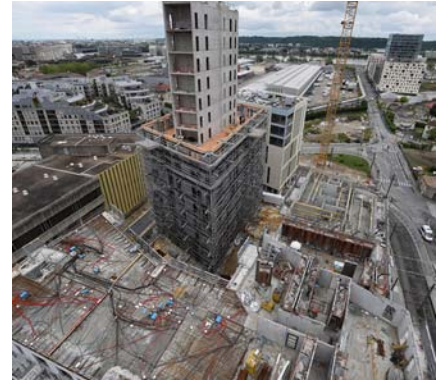
Aerial view of the construction process. David Sebastián Martín
