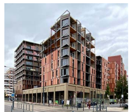
Construction of the facade of the dwellings using prefabricated panels.
