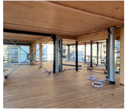
Mixed timber-steel structure and cross bracing system. ICADE
