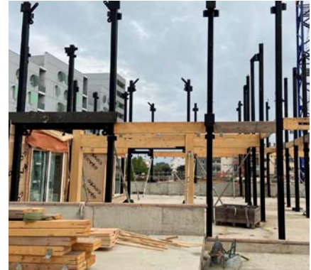
Mixed timber-steel structure . ICADE
